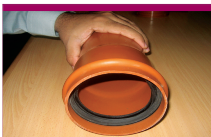
Make sure that the rubber ring is firmly in the socket with no edges out of the ring groove
